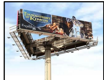
CENTER MONOPOLE TRI-SIDED
