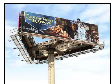
CENTER MONOPOLE TRI-SIDED
