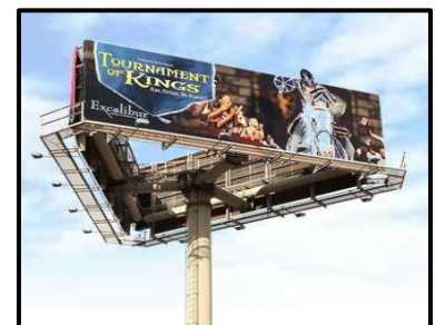
CENTER MONOPOLE TRI-SIDED
