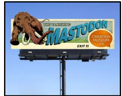
CENTER MONOPOLE DOUBLE FACE
